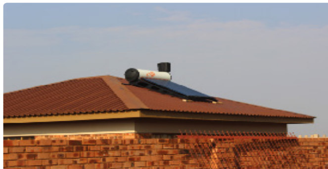
Solar hot water heating system on roof
