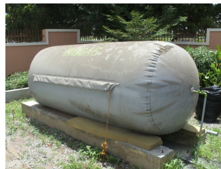
Above ground plastic inflatable gasholder
