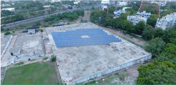
The 145 kW Solar PV system installed at one of Rajkot's water treatment plant, as part of its Urban-LEDS response in phase 1
