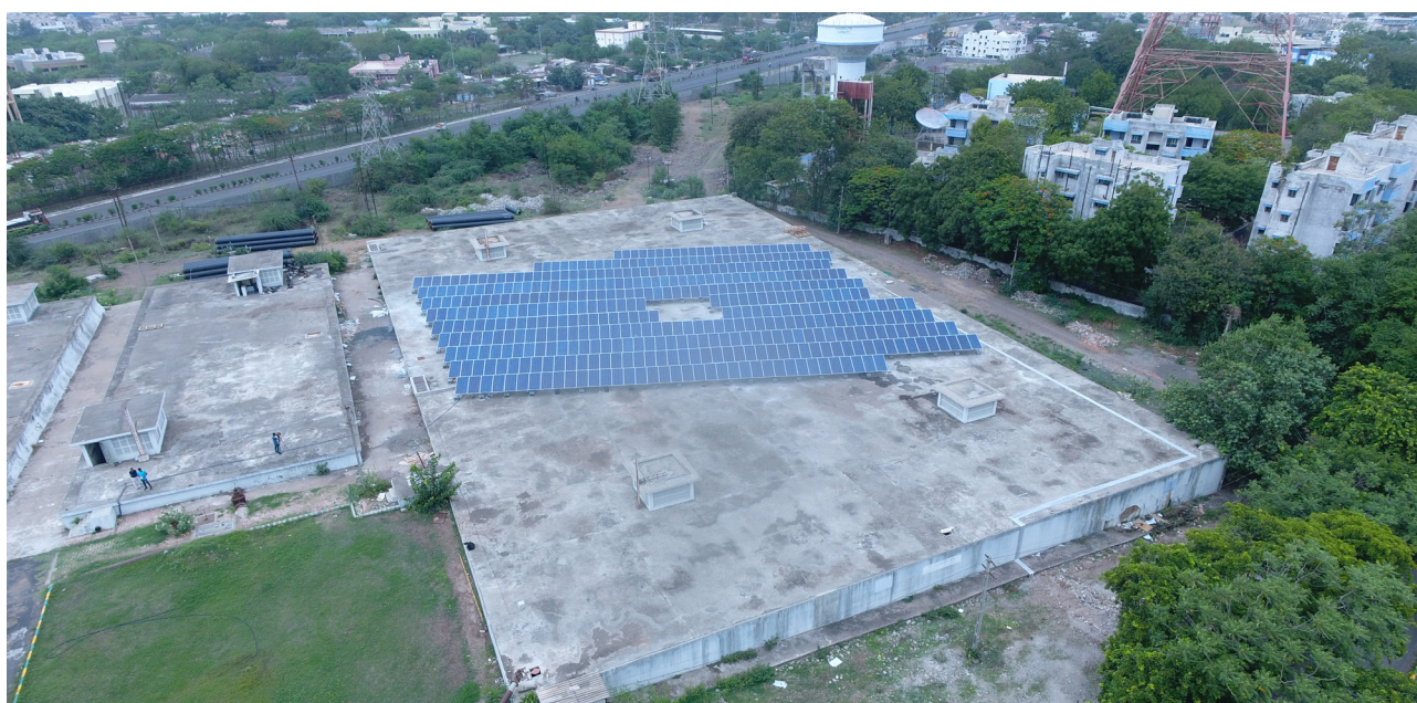
145-kilowatt solar PV system installed at the Aji Water Treatment Plant, Rajkot © Rajkot Municipal Corporation
