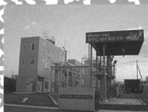
Kyoto city BDF plant
